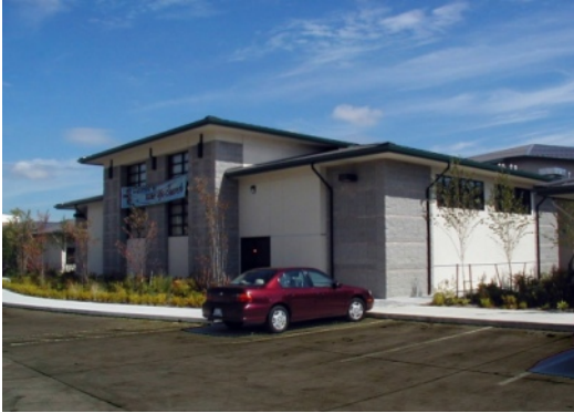
Phase II Addition
