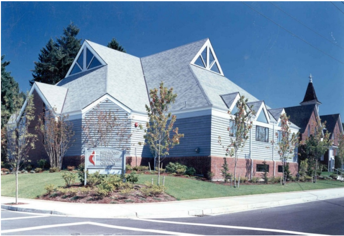
View at Sanctuary Exterior
