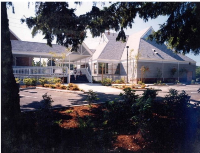
Exterior View of Covered Connection and Ramps
