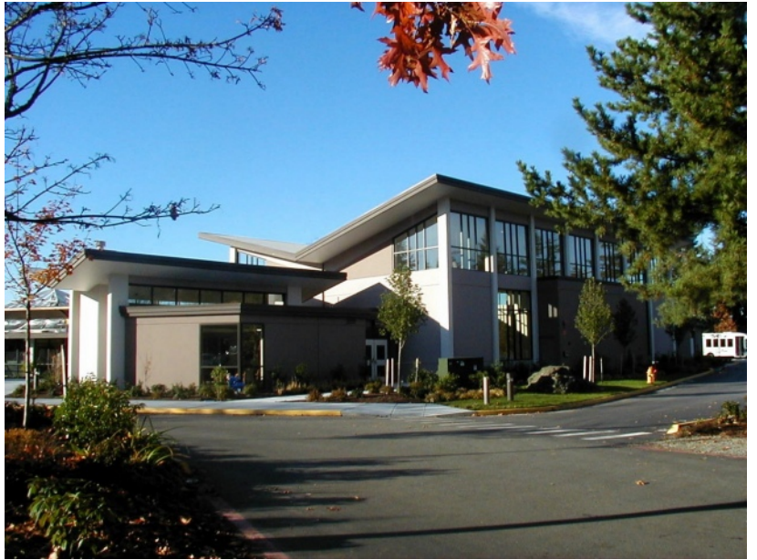
Exterior View of Multi-Use Room
