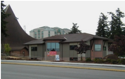
Exterior View from Street
